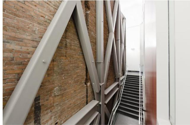
Figure 2. Structural steel seismic bracing – Canadian Museum of Nature, Ottawa. [3]
